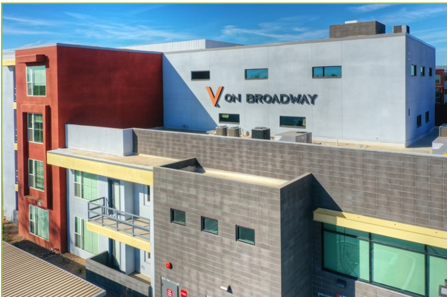
The 90-Unit Broadway Apartments in Tempe
